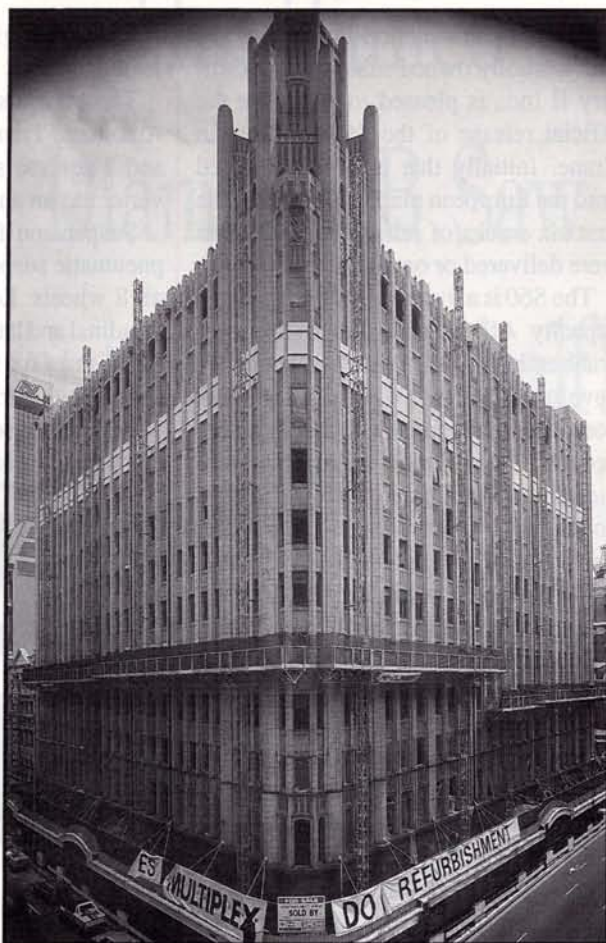
Hi-Climber units are being used by Multiplex in the refurbishment of the historic Grace Building in Sydney.
